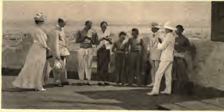
JOINING THE P.T.L. ON TOP OF THE WATER TOWER AT HANKOW, SEPT. 1909.
